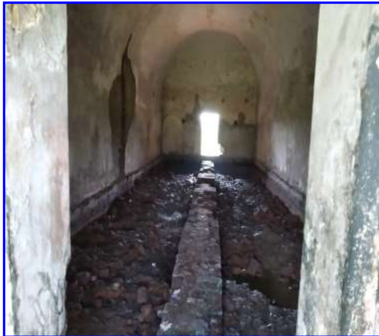
Fig. 6. BAROOD GHAR – The gunpowder was stored beneath this floor, as the public says
